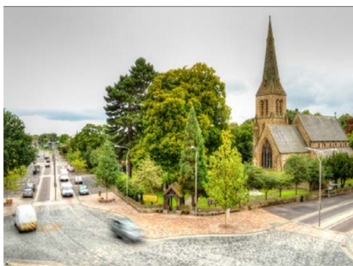
Roundal Junctions - better manage turning traffic, creating slower but steady pace and improved pedestrian crossing
